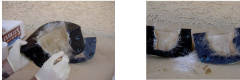
Figure 34 & 35: Detail of Resin Application
