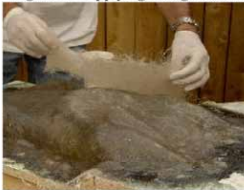
Figure 22: Applying fiberglass mat
