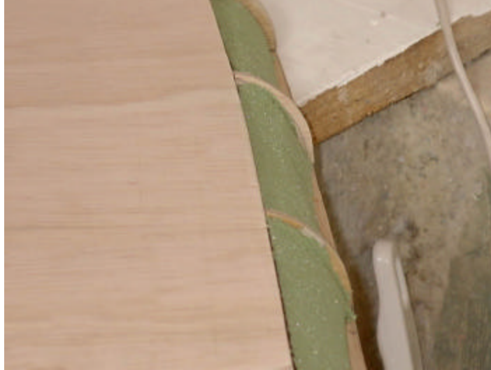
Figure 20: Removing Foam for Bondo Application
