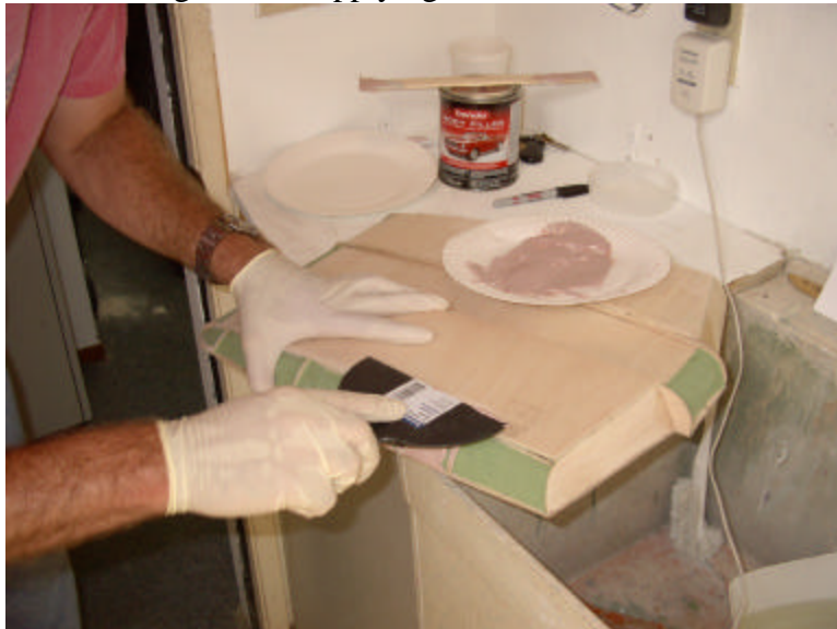
Figure 21: Applying Bondo Over Foam
