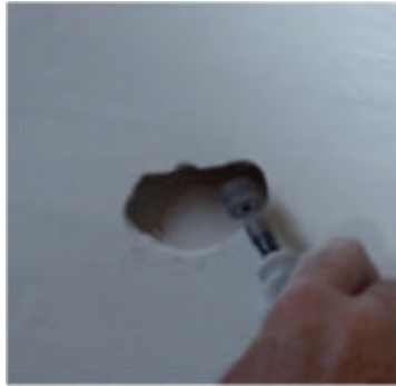
Figure 11 Beveling the Repair
