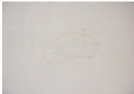
Figure 26 Repair is Semi-Finished
