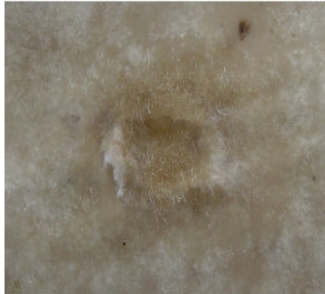
Figure 25 the finished repair from the inside surface
