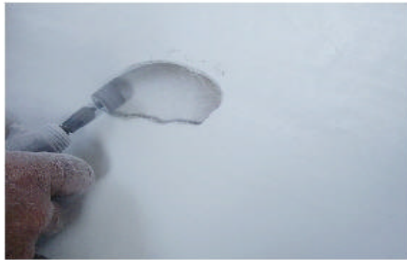
Figure 10 Damaged Area Removed
