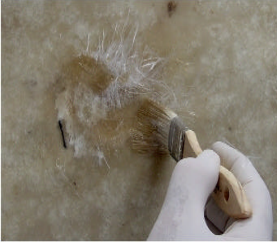
Figure 24 Finishing the mat application
